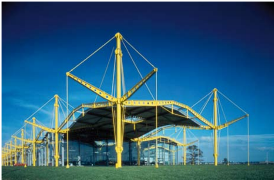
Figure 2.14 Suspended structure used at the Renault Factory, Swindon, UK built in the 1980's Architect: Richard Rogers Partnership
