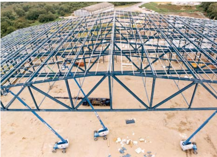
Figure 2.11 (Above) Various forms of lattice truss used in industrial buildings
