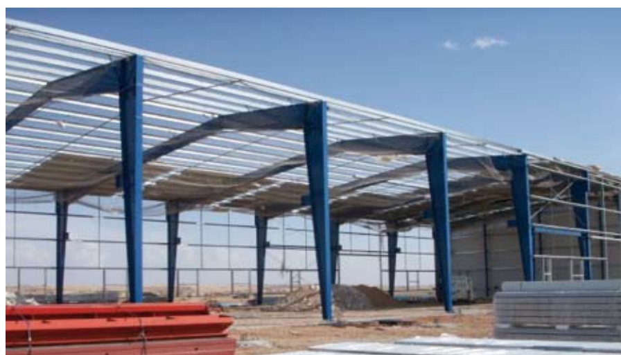
Figure 5.9 Single portal frames with tapered columns and rafters under construction in Spain
