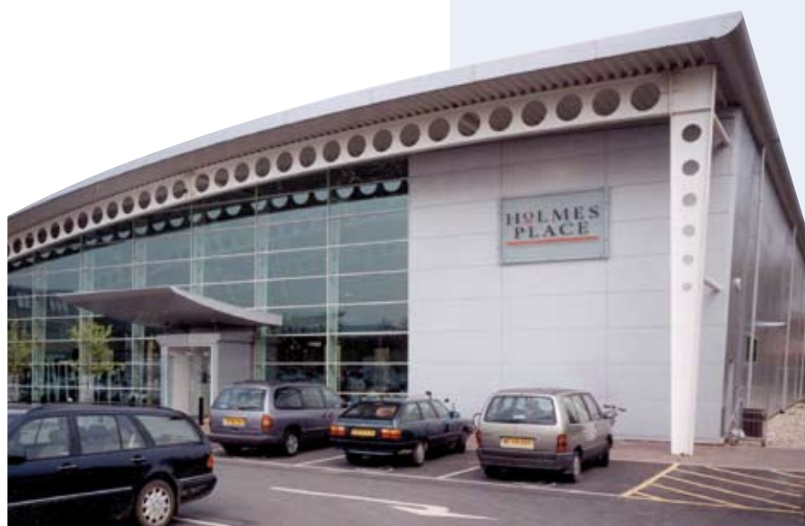
Figure 1.1 Leisure building using a steel framed structure
