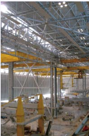
Internal view of the building during construction
